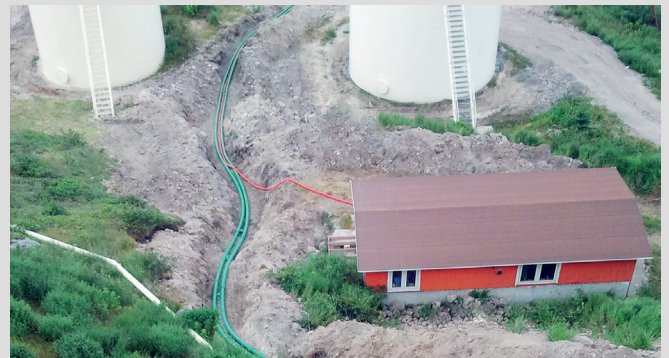
EDF Thermal Power Plant, Saint Pierre, France
